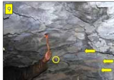
Figure 8: Low arched roof with little collapse.
